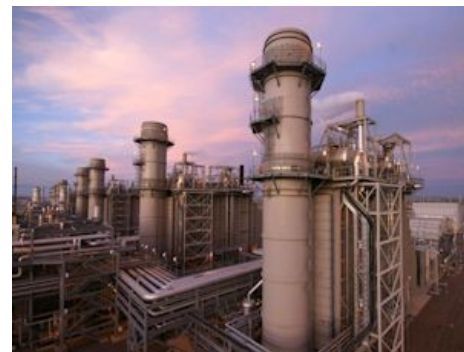
Union Power combined cycle plant Source: Entergy
