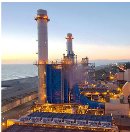
El Segundo gas plant in California Source: NRG Energy
