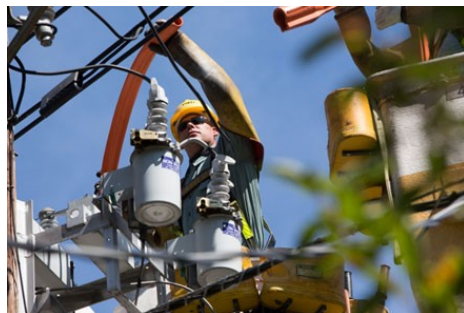
PSE&G line workers perform upgrades Source: PSE&G
